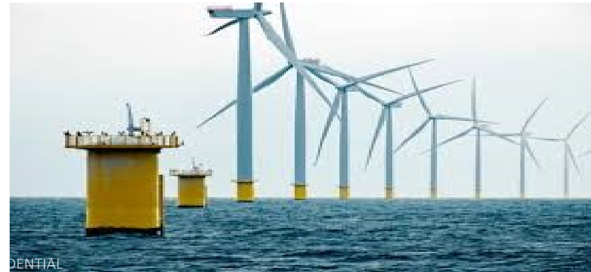
Figure 1. Typical Monopile Wind Turbine (left) and Mini Jacket type Wind Turbine (right).
