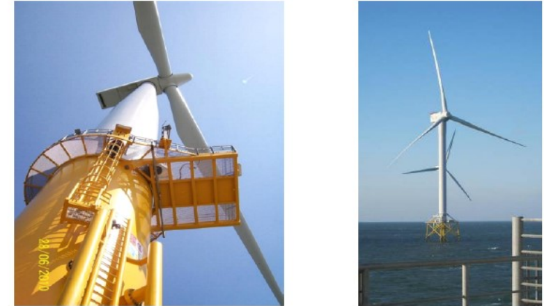
Figure 1. Typical Monopile Wind Turbine (left) and Mini Jacket type Wind Turbine (right).
