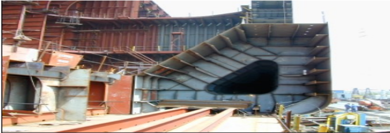
Fig. A5 View of Hopper After Erection, Looking Aft
