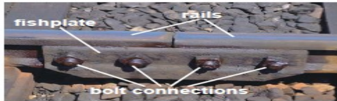
Fig. 1. Bolted rail joint components
