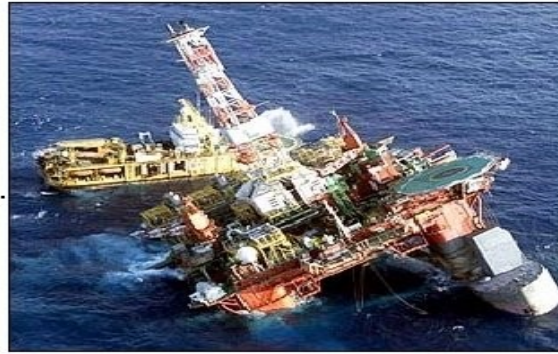
Recent (2001) failure of offshore oil platform near Brazil
